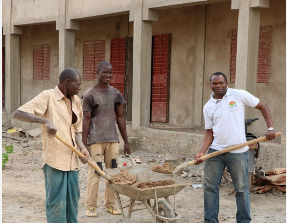
Alfred helping at the school construction site in Burkina Faso
