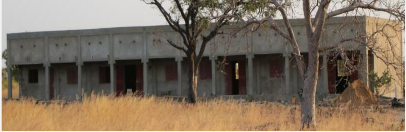
The school first wing on the finishing phase.
