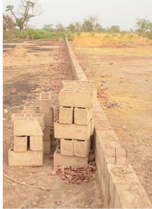
School wall under construction.
